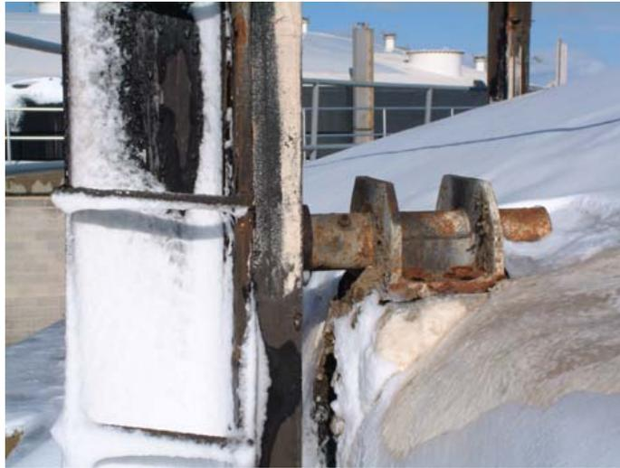
**Figure 2. Roller Guide Installed On Cover**
