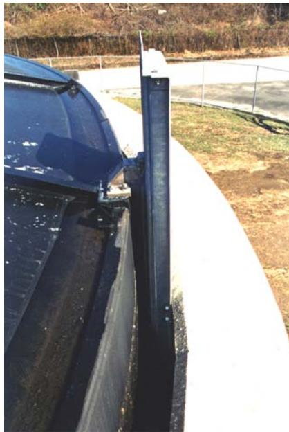
**Figure 8. Full-length Slide Guide Installed in Digester Cover**
