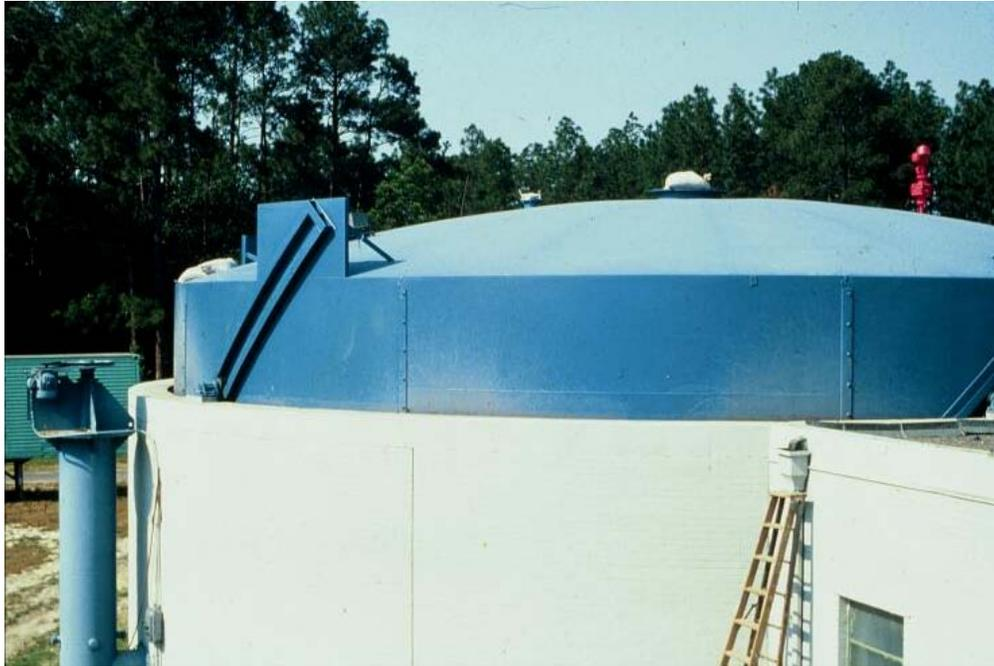
**Figure 4. Spirally Guided Digester Cover with Rollers**
