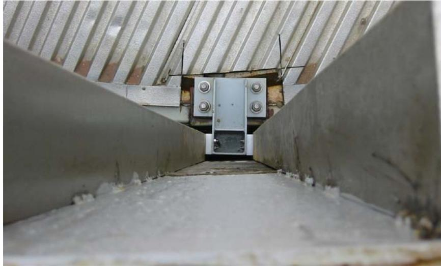
**Figure 7. First Generation Slide Guide**
