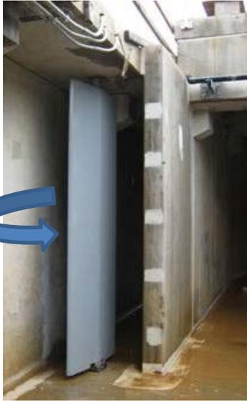
Placed at the entry to the internal recycle (IR) channel, the Eliminat<sup>IR</sup> gate replaces expensive IR pumps and older manual gates. Either the center pivot or the end pivot (common for manual IR gates currently installed) designs are available.
