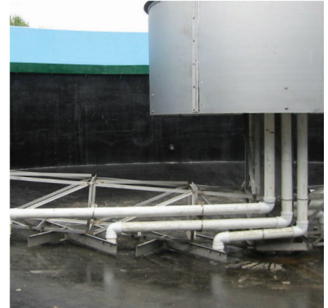
SUCTION TUBE CONFIGURATION
