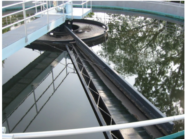
FULL TROUGH SKIMMER (FTS) SYSTEM SYSTEM
