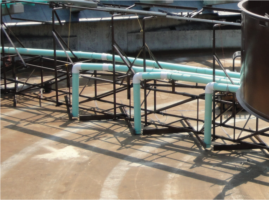
SUCTION TUBE CONFIGURATION
